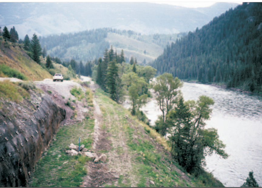
Completed soil nail wall with temporary rock-fall mesh facing, prior to installation of a segmental block MSE retaining wall.
