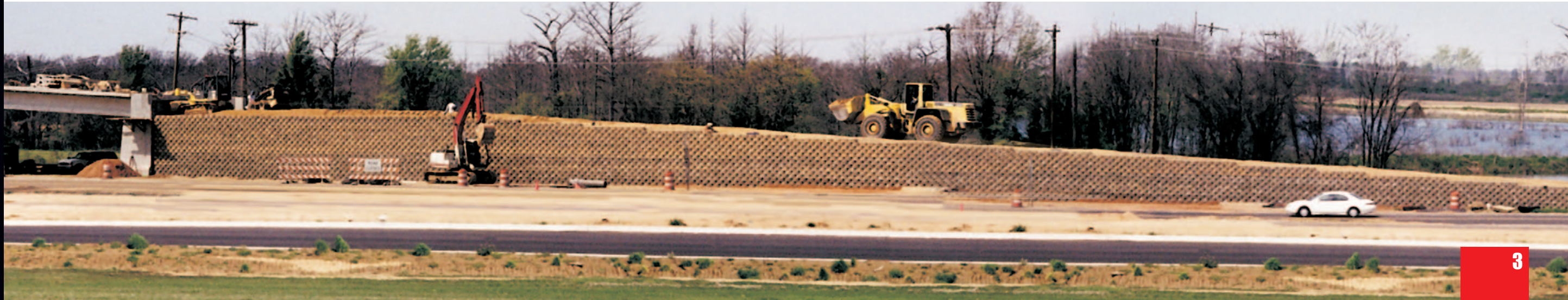
Mississippi Department of Transportation - Yazoo City, MS 13,200 s.f. segmental block MSE retaining wall bridge lead up ramps
