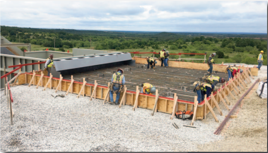
Prefabricated steel bump curb and reinforced concrete approach slab
