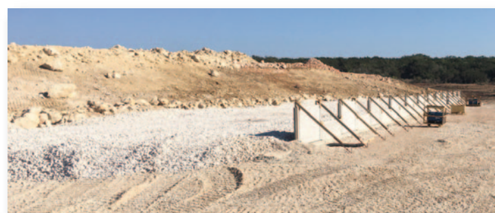
Aggregates Mine - Hondo, Texas 10,000 s.f. precast concrete panel MSE retaining wall dump structure and 900' lead up ramp, 50' tall
