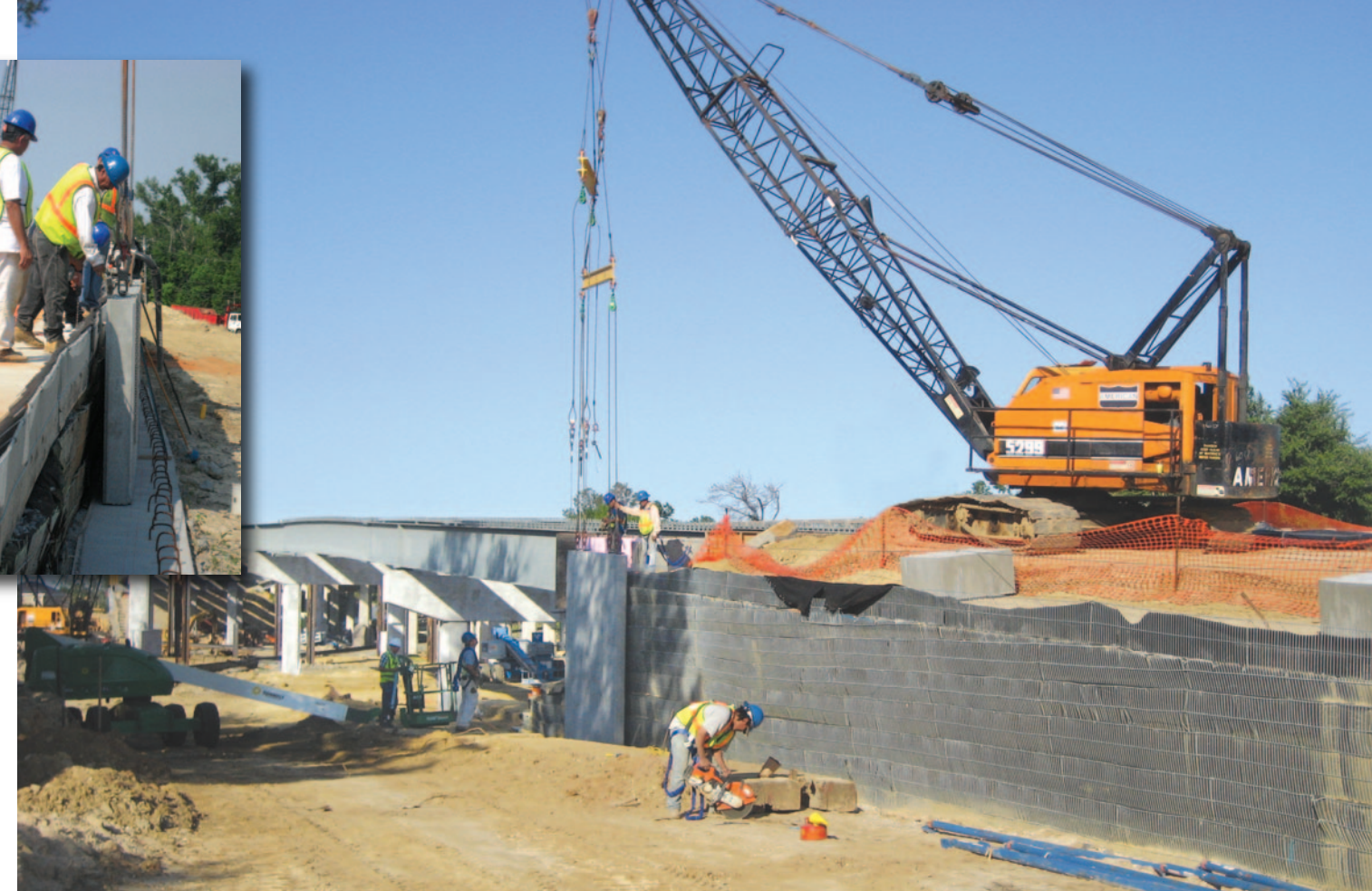
2-stage welded wire MSE retaining wall with full-height precast concrete panels.
