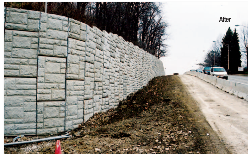
Sam's Club - Cuyahoga Falls, Ohio 8,000 s.f. rock anchor assisted precast concrete panel MSE retaining wall
