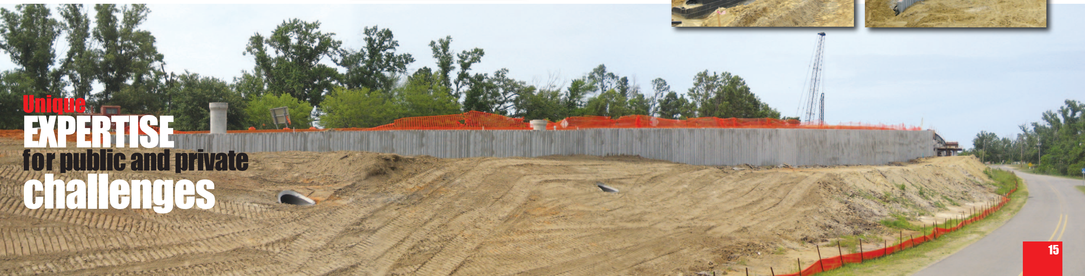
Mississippi Department of Transportation - Biloxi, MS and Pass Christian, MS 17,000 s.f. and 3,000 s.f. 2-stage MSE retaining wall bridge lead up ramps with full-height precast concrete panels. (Two of the many bridge structures rebuilt after Hurricane Katrina.)
