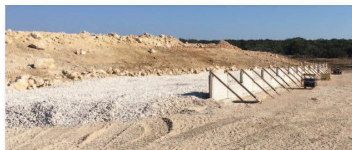
Aggregates Mine - Hondo, Texas 10,000 s.f. MSE dump structure and 900' lead-up ramp, 50' tall
