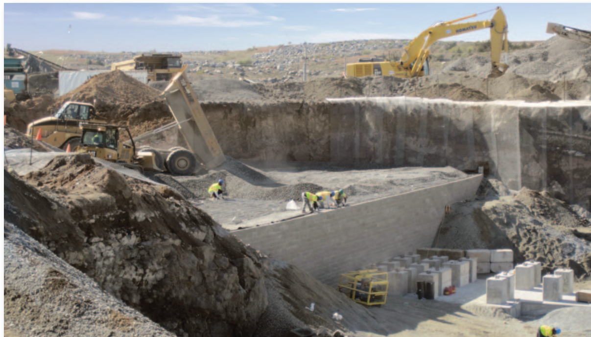
Aggregates Mine and Manufacturing facility - Roosevelt, Oklahoma 5,000 s.f. MSE dump structure, 38' tall Permanent fall-protection and dump curb system Simultaneous installation; MSE dump structure and primary crusher
