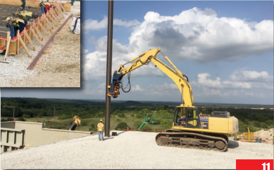
Steel H-piles installed with 100 ton high-frequency vibro hammer
