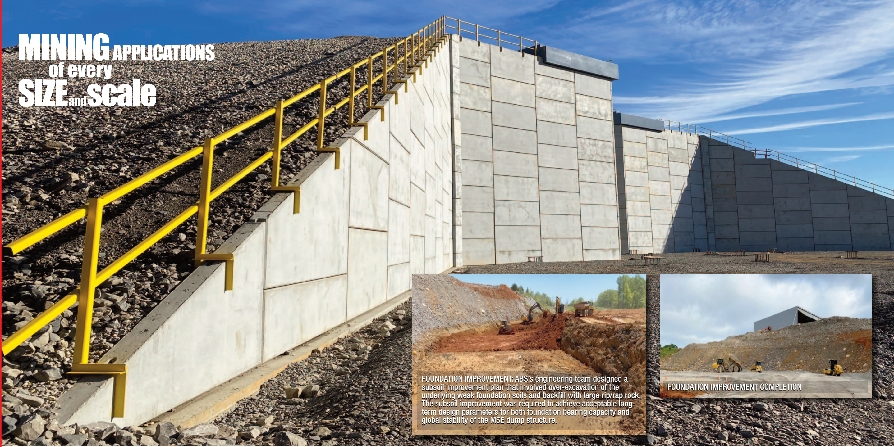
Aggregates Mine, Cement Manufacturing Facility - Mitchell, Indiana 11,000 s.f. MSE dump structure and lead-up ramp, 50' tall Permanent fall-protection system and SafTcurb™ engineered dump curb system
