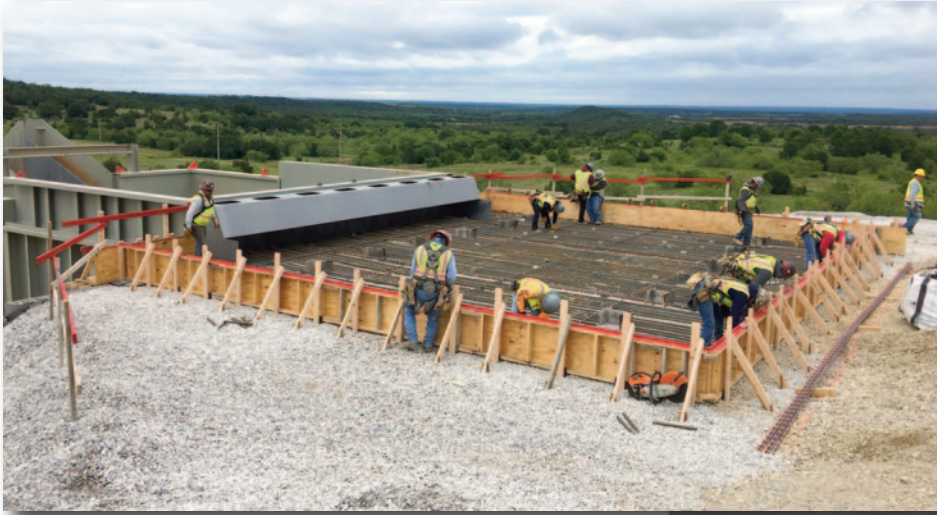
Dump curb and reinforced concrete approach slab installation
