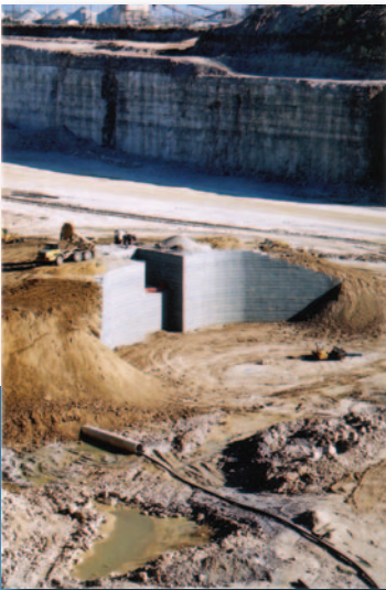
Hanson Aggregates Mine - Chico, Texas 13,000 s.f. MSE dump structure and lead-up ramp, 50' tall
